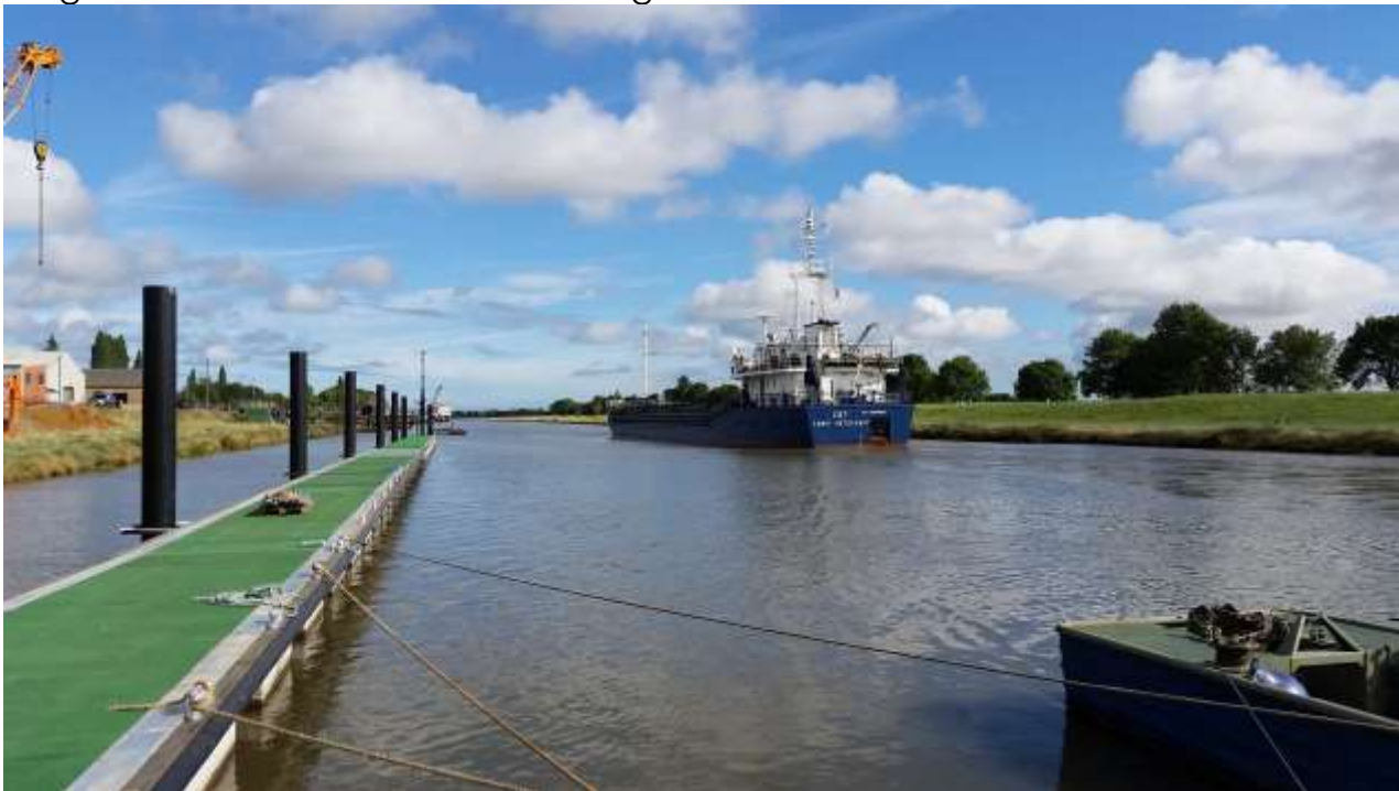
Progress Photo – Commercial Moorings
