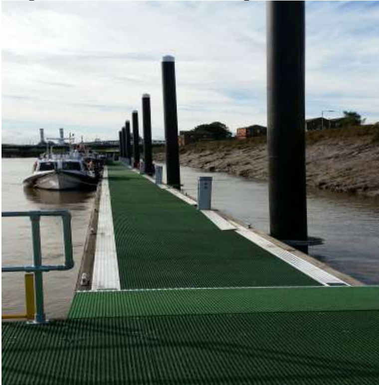
Progress Photo – Leisure Moorings
