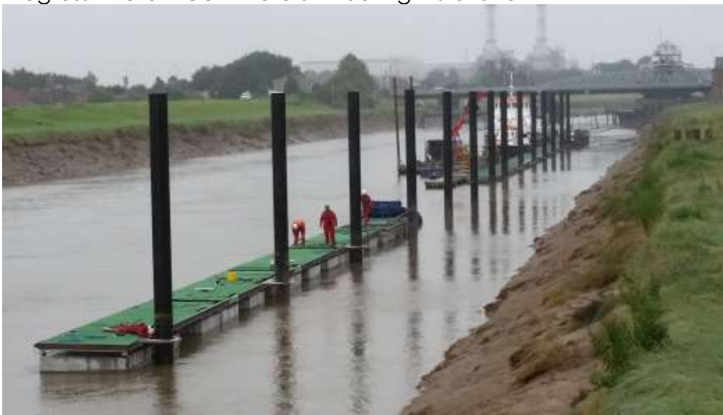
Progress Photo – Commercial Mooring Installation
